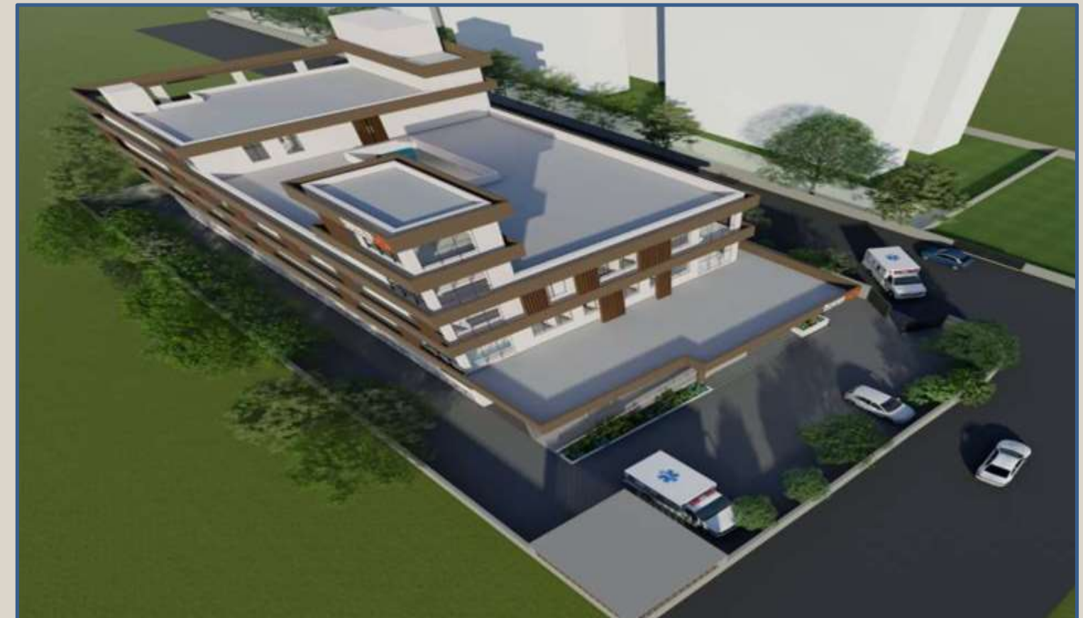
VINAYAK HOSPITAL, UNDRI, PUNE
