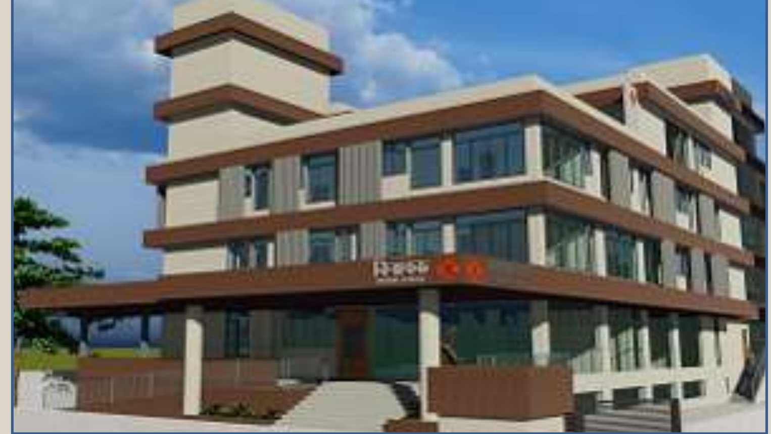
VINAYAK HOSPITAL, UNDRI, PUNE
