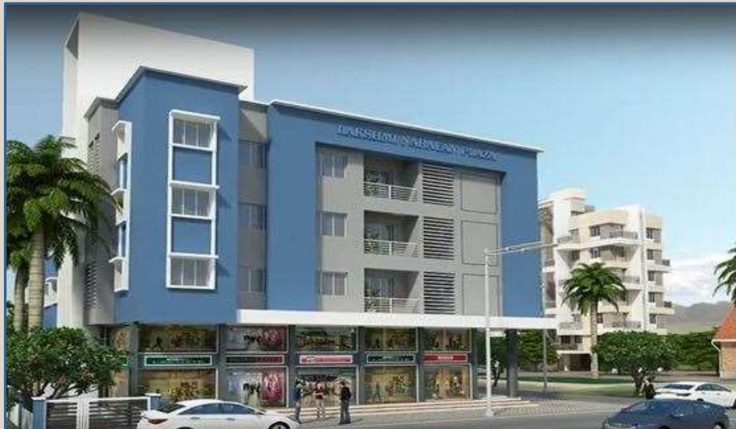
LAXMI NARAYAN COMPLEX, GOREGAON, RAIGAD
