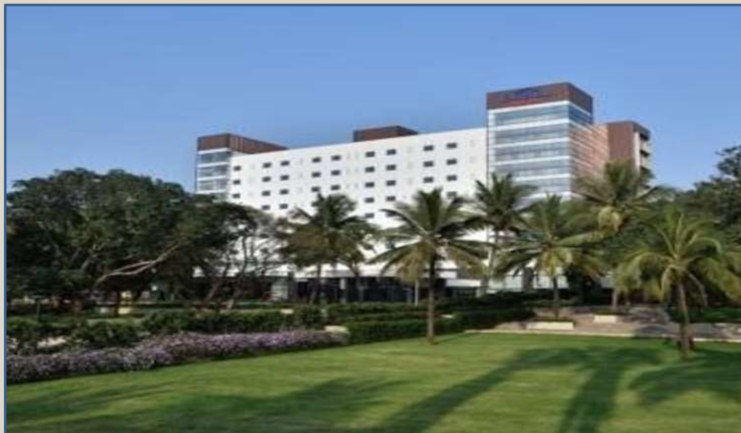
FAIRFIELD MARRIOTT, BELAGAVI
