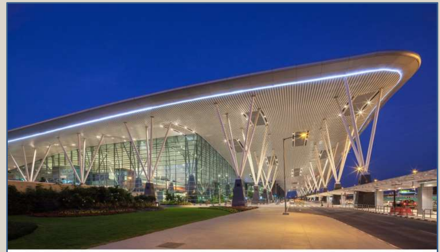
BENGALURU INTERNATIONAL AIRPORT
